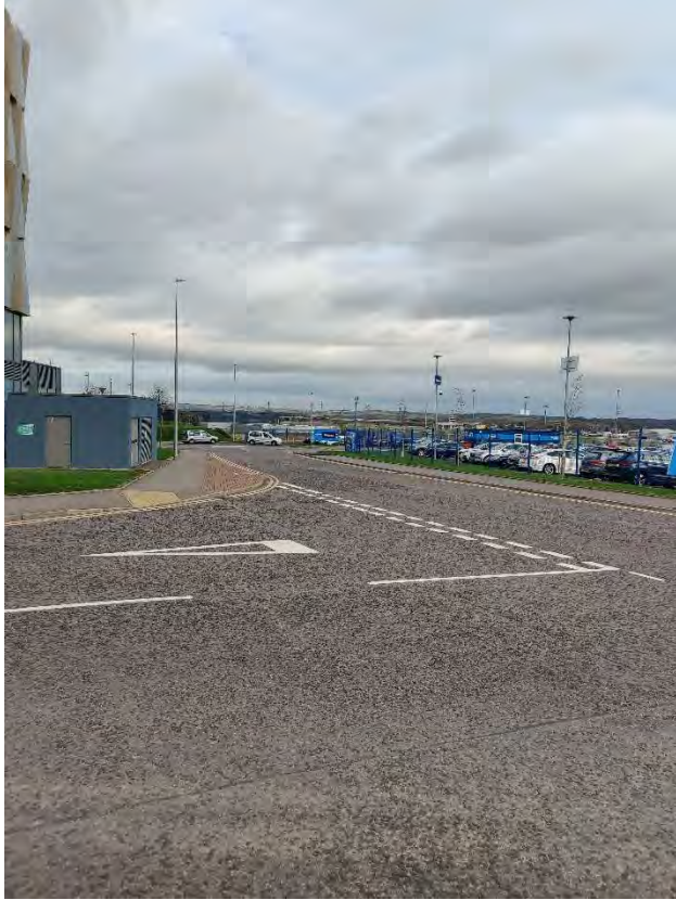
Argyll Way / International Way Junction
