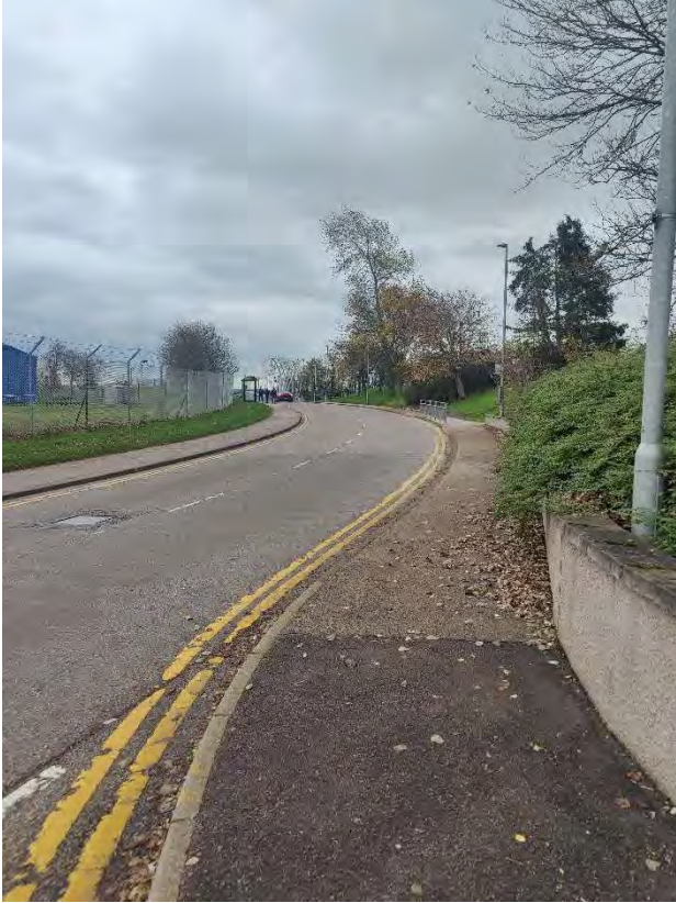
Forties Road (Eastbound)
